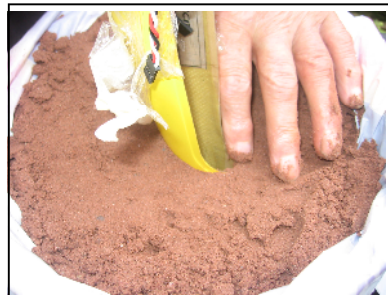
Compacting the sand round the nose to make a pattern to pour the molten lead in
